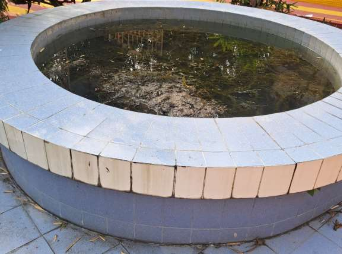
Rain water storage
